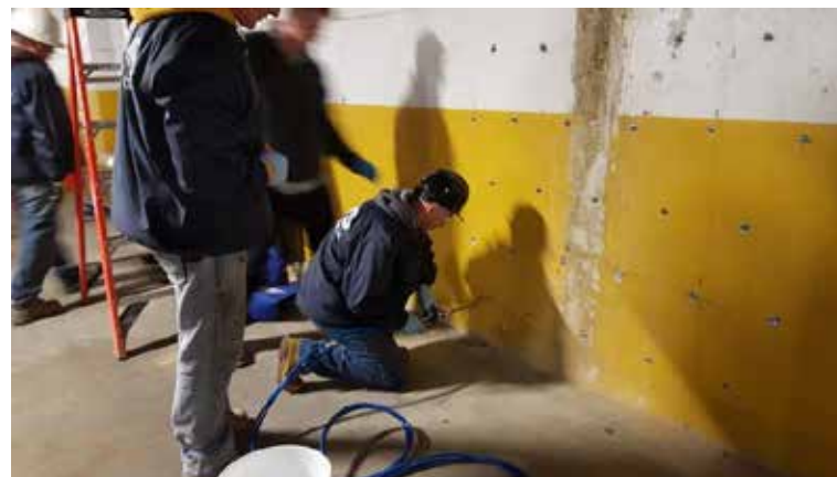
Injection of gel through ports (packers)
