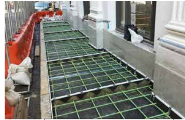
Reinforcement install
