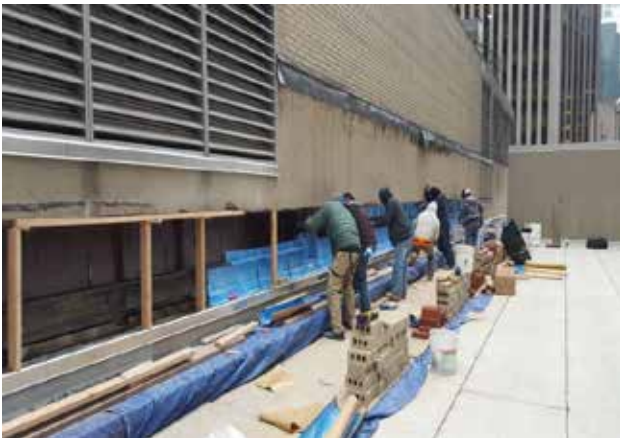
Spandrel beam rehabilitation and waterproofing
