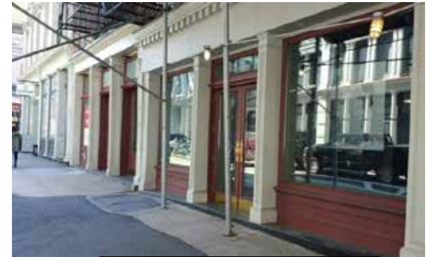
Finished storefront install View 2
