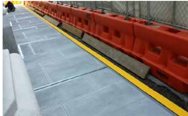
Finished sidewalk & vault
