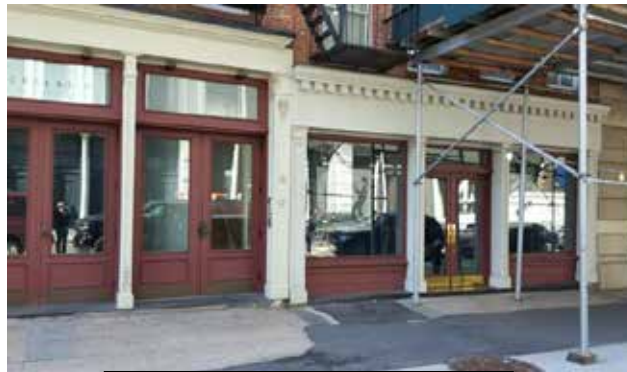
Finished storefront install View 1
