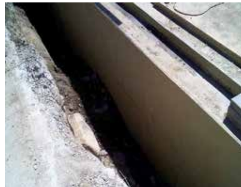
Foundation wall prep.
