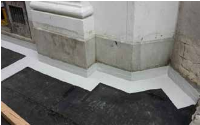
Parapro base flashing
