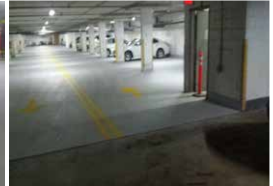
Finished with line striping
