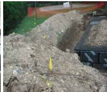
Waterproofing install
