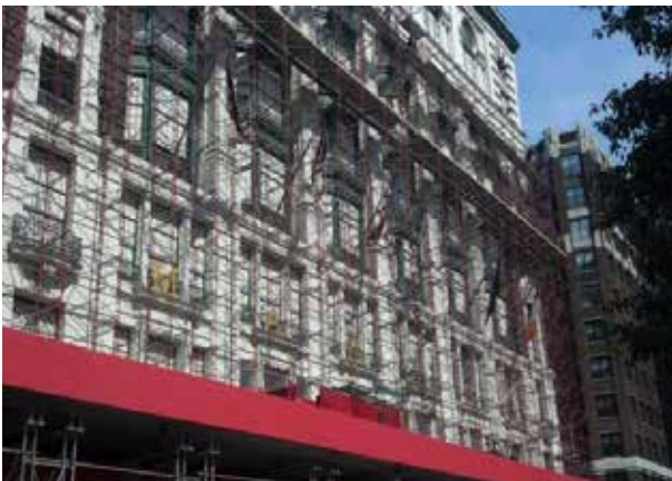
Sidewalk bridge and pipe scaffold erection
