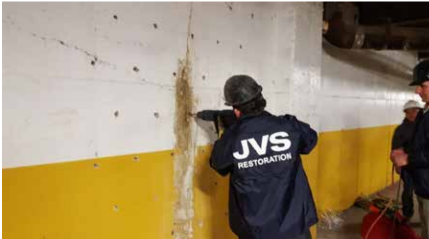
Prep for gel injection drilling of thru-wall holes
