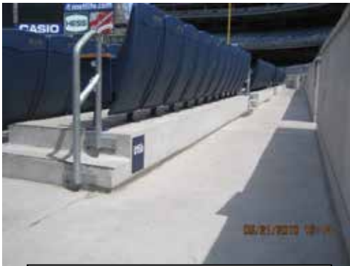
Stadium expansion joint condition
