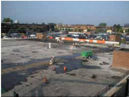
Membrane removal process
