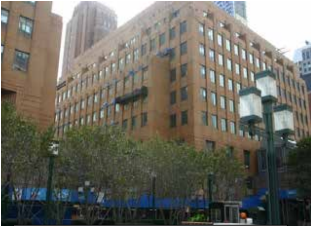
Rigging for shelf angle and sealant replacement
