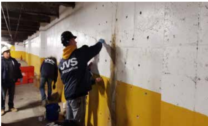
Insertion of injection ports (packers) hand tightened with wrench
