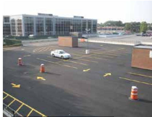
Finished asphalt with line striping
