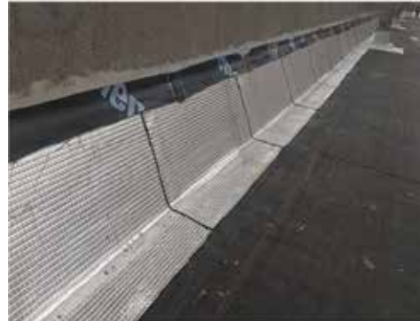
Siplast veral aluminum flashing install
