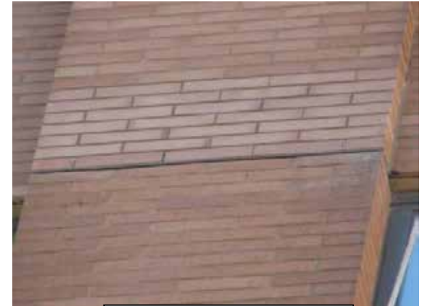
Finished masonry brick install
