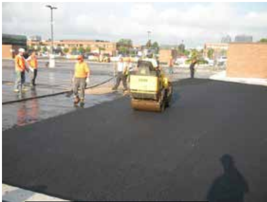
Asphalt install
