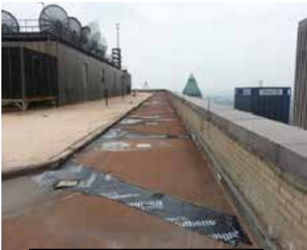
Existing waterproofing condition
