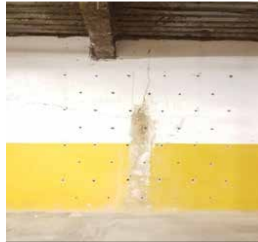
Completed thru wall 5/8" holes drilled at a 12" O.C. pattern
