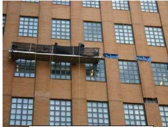
Column shelf angle rehabilitation shelf
