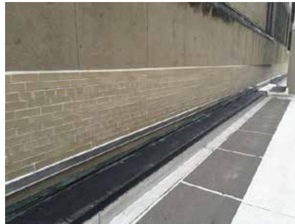
Finished brick masonry and aluminum flashing
