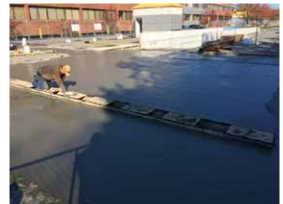
Expansion joint & concrete install
