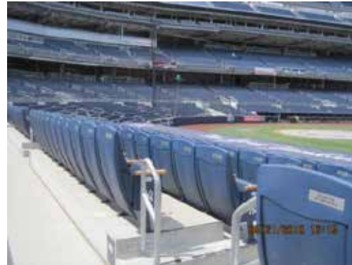
New DSM expansion joint install
