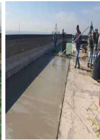
New concrete installation
