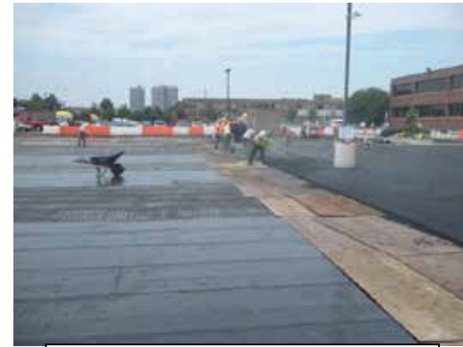
Asphalt install with membrane protection
