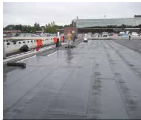
Siplast Teranap membrane install
