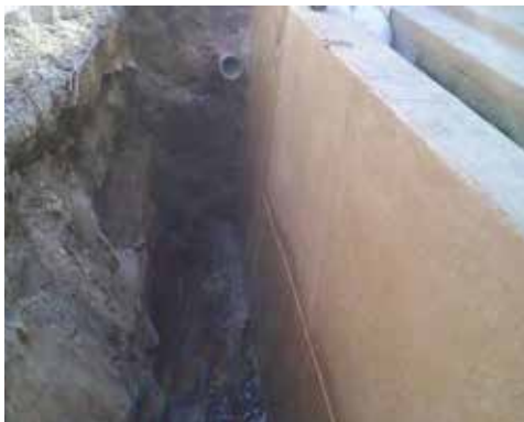
Excavation of foundation wall
