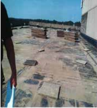
Existing overburden and membrane
