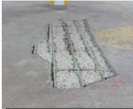
Preparation with new reinforcement
