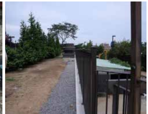
Coping stone installed and draining ground
